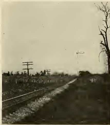
FIG. 6. SIGNAL ARM HORIZONTAL, BLOCK OCCUPIED; STOP.
